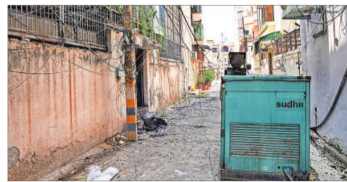
BACK LANE TOO NARROW: The lane behind the building is too narrow for a fire truck to enter. Fire personnel tried to break through the grills to enter the flat. One resident got a mechanised iron cutter, operated with a power generator.
