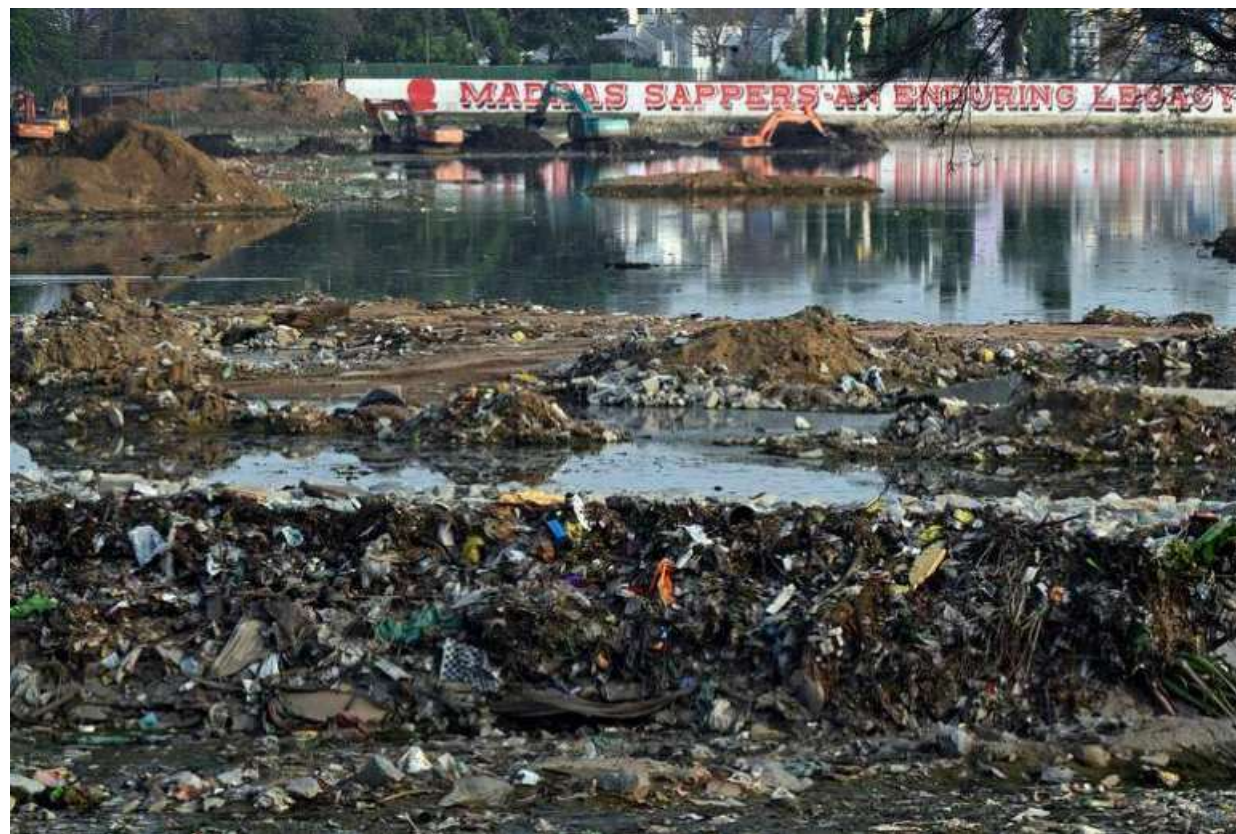
Restoring glory: Desilting work is under way at Ulsoor Lake in Bengaluru on Thursday, as part of a ₹107-crore rejuvenation project for the 106-acre water body, one of the few in central Bengaluru. SUDHAKARA JAIN
