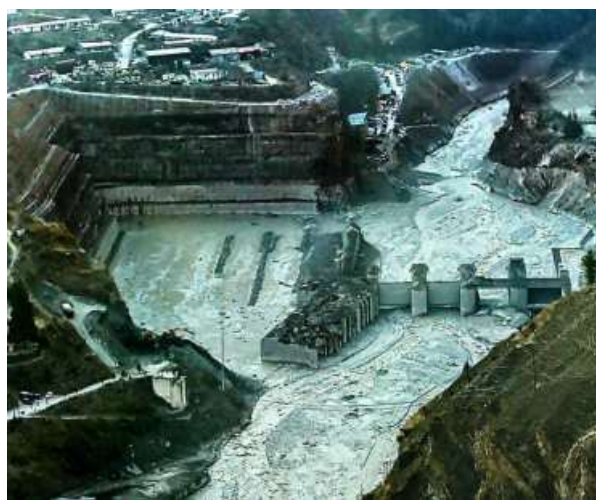
The Tapovan hydel power project was damaged during the 2021 Rishiganga flood in Chamoli district of Uttarakhand. PTI
