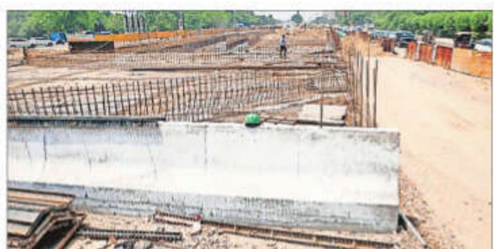
Construction work underway at Gaur Chowk. GAJENDRA YADAV
