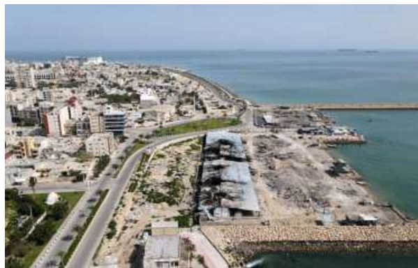
Locked and loaded: Damage at a fishing pier, reportedly due to the U.S.-Israeli air strikes, in the port of Qeshm island in Iran. AP
