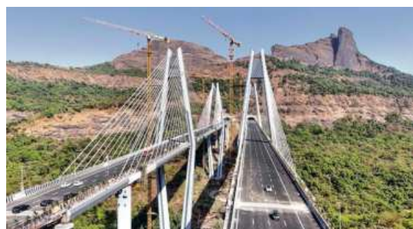
The Mumbai-Pune Expressway 'Missing Link' project is seen on the day of its inauguration, in Mumbai, Maharashtra on Friday. PTI
