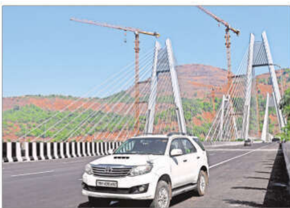
The 'Missing Link' project includes two tunnels, two viaducts and a cable-stayed bridge over Tiger Valley. DEEPAK JOSHI
