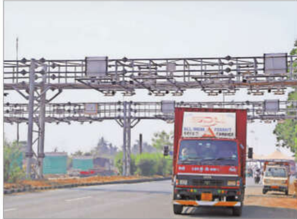
The MLFF system works without a boom barrier and vehicles are not supposed to stop for toll payment. EXPRESS
