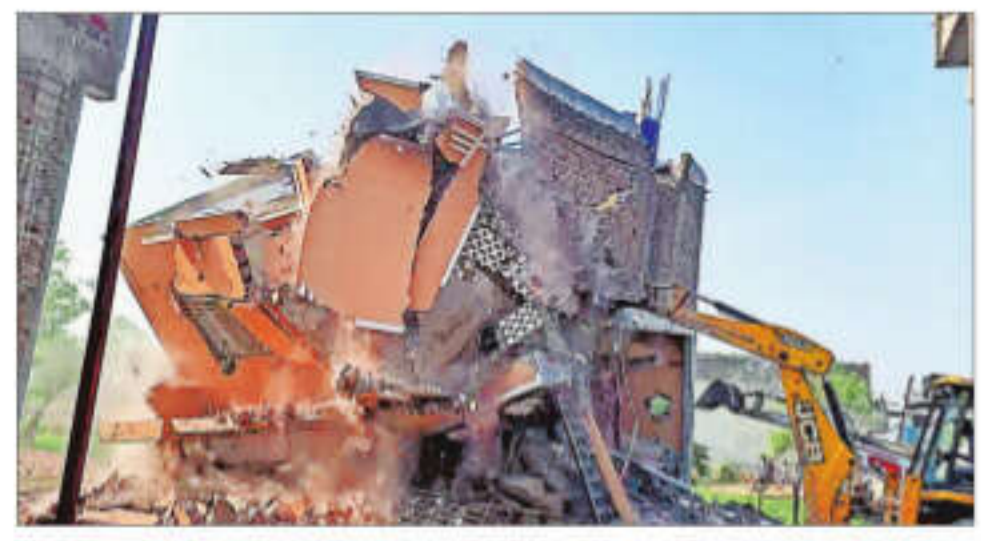
Demolition underway in Chhatrapati Sambhaji Nagar, Wednesday. ANI
