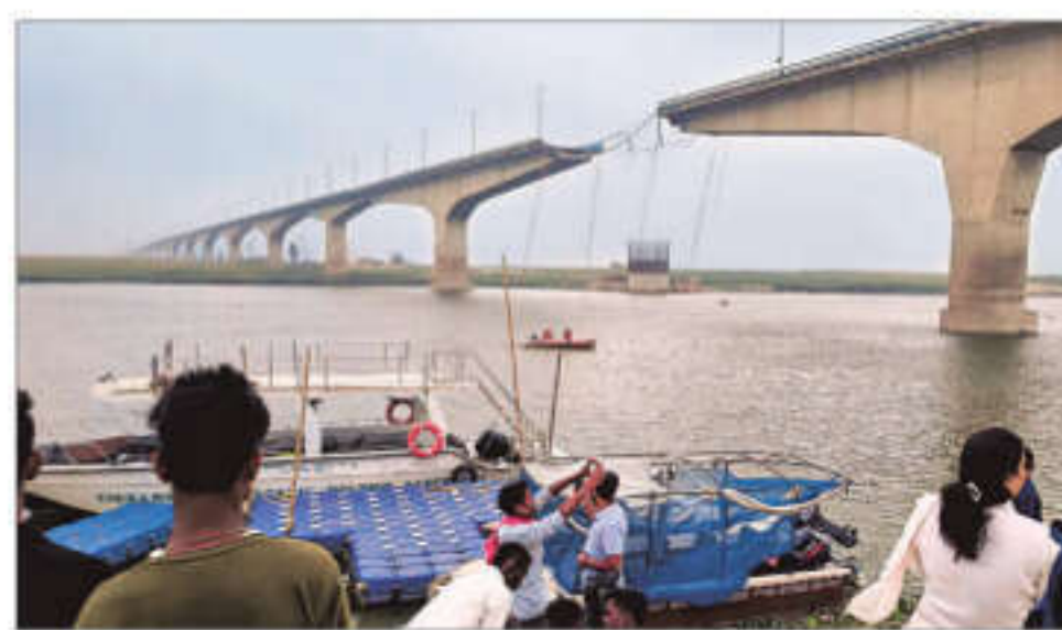
A portion of the Vikramshila bridge collapsed last week. EXPRESS
