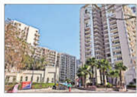
Indiabulls Centrum Park, Sector 103 off Dwarka Expressway
