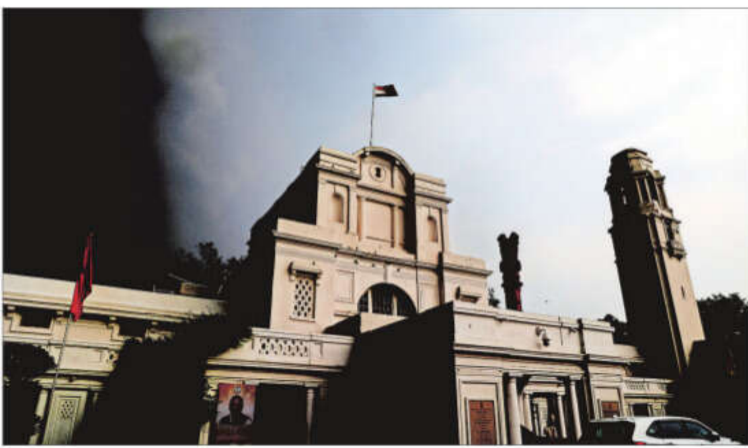
3:15 PM View of the Delhi Vidhan Sabha after rain and a dust storm struck the Capital. AMIT MEHRA
