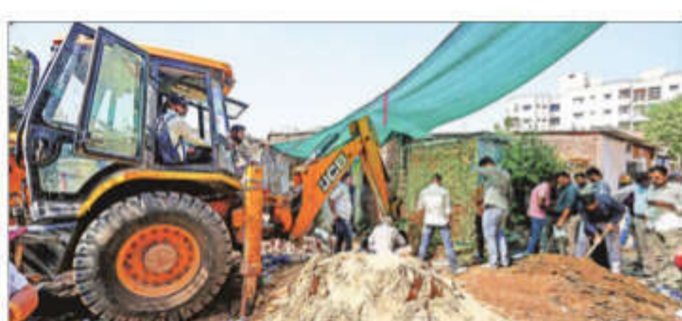
An excavator on the premises of the house, Wednesday. BHUPENDRA RANA
